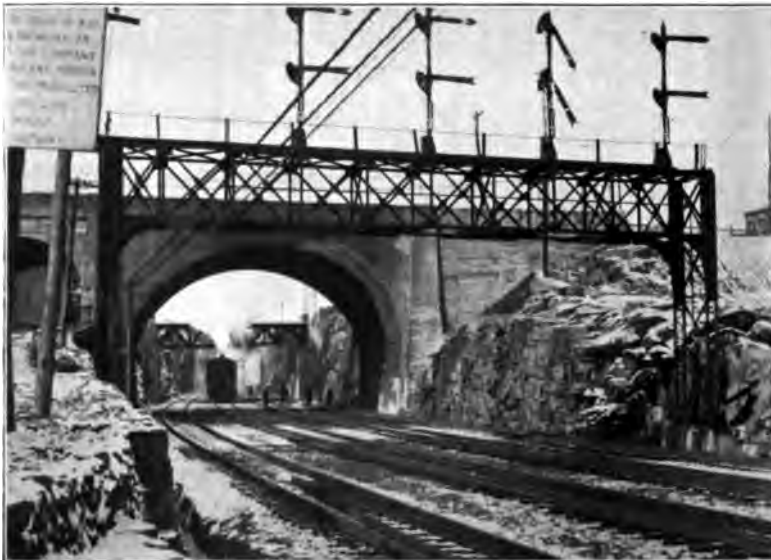
ENTRANCE TO THE GREAT FOUR-TRACK OPEN CUT WHICH THE ERIE HAS BUILT FOR THE COMMUTER'S COMFORT AT JERSEY CITY -
